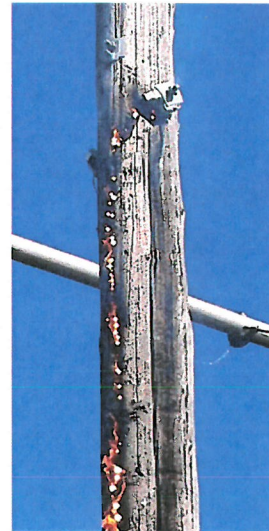
Figure 2 – Treated Wood Pole Burning
