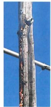
Figure 2 – Treated Wood Pole Burning
